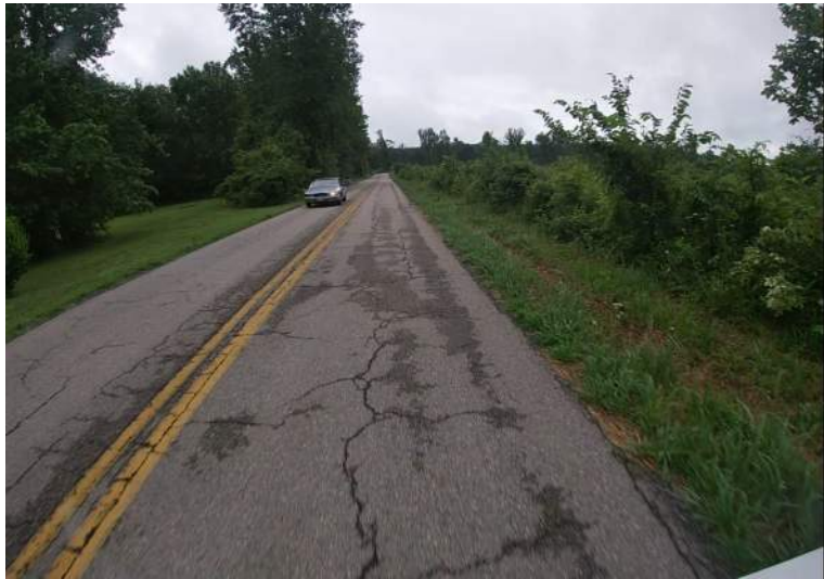
8. Block Cracking
