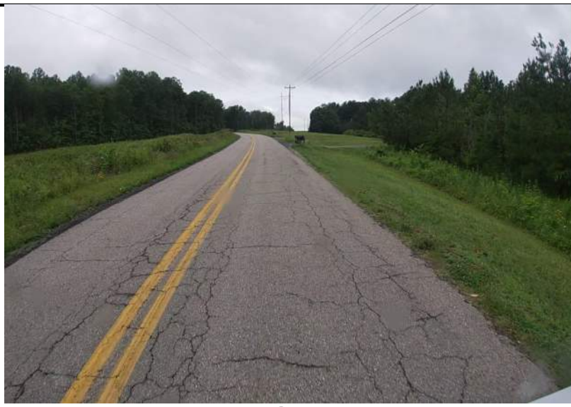
19. Block Cracking
