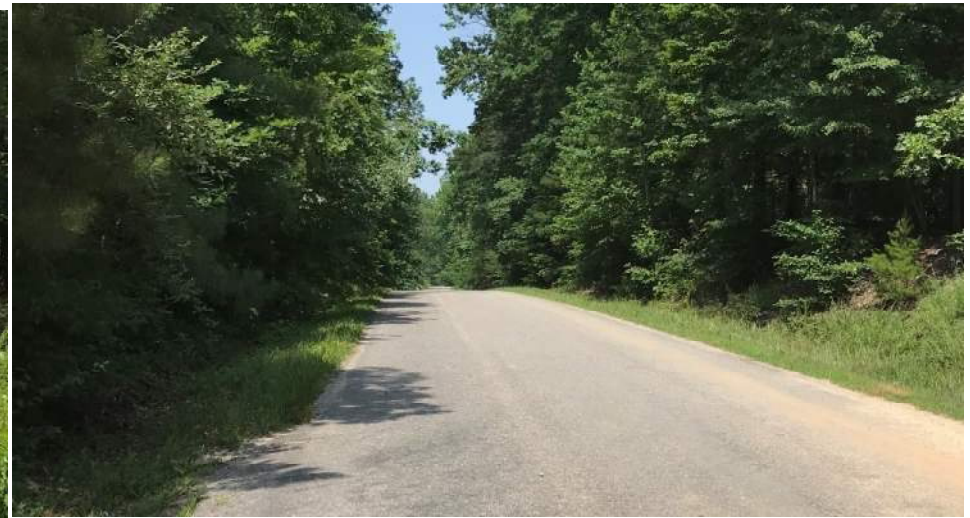
East along Route 609
