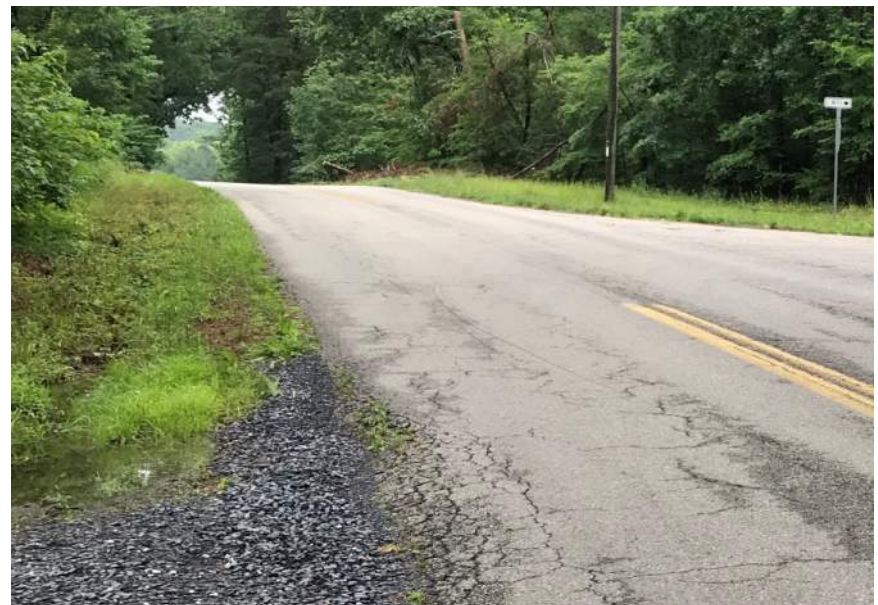
East along Route 690
