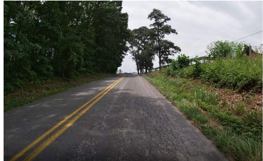
36. Alligator Cracking
