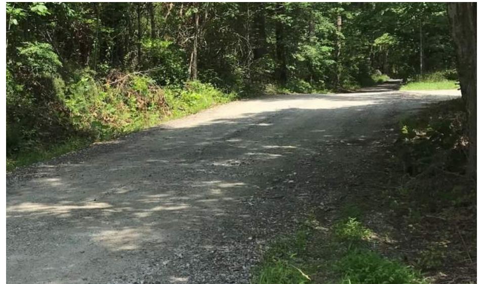
North along Route 608
