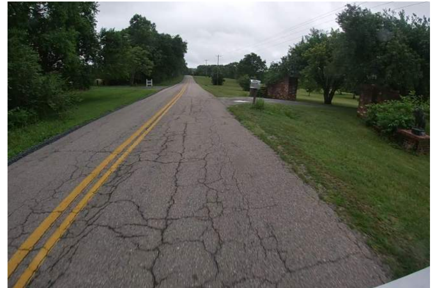
14. Alligator Cracking
