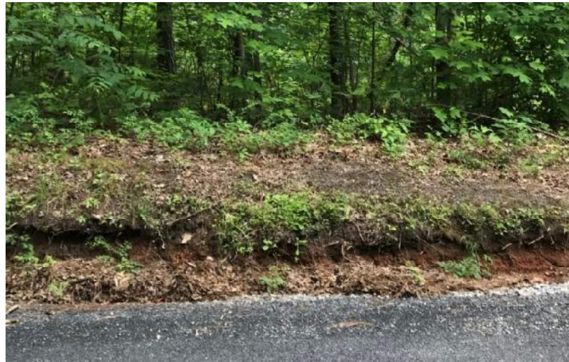
South along Site Entrance
