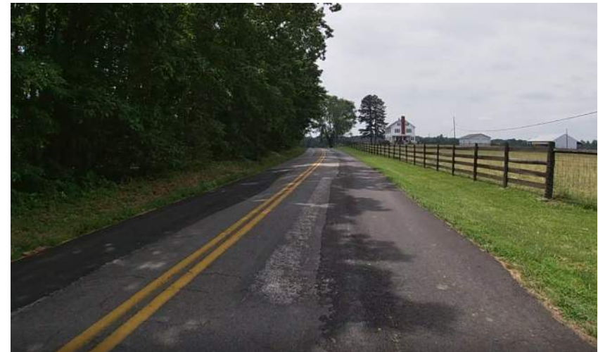
36. Alligator Cracking
