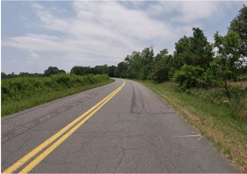
13. Block Cracking, Patching
