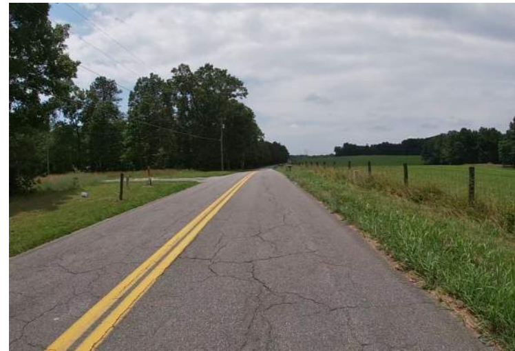
30. Block Cracking
