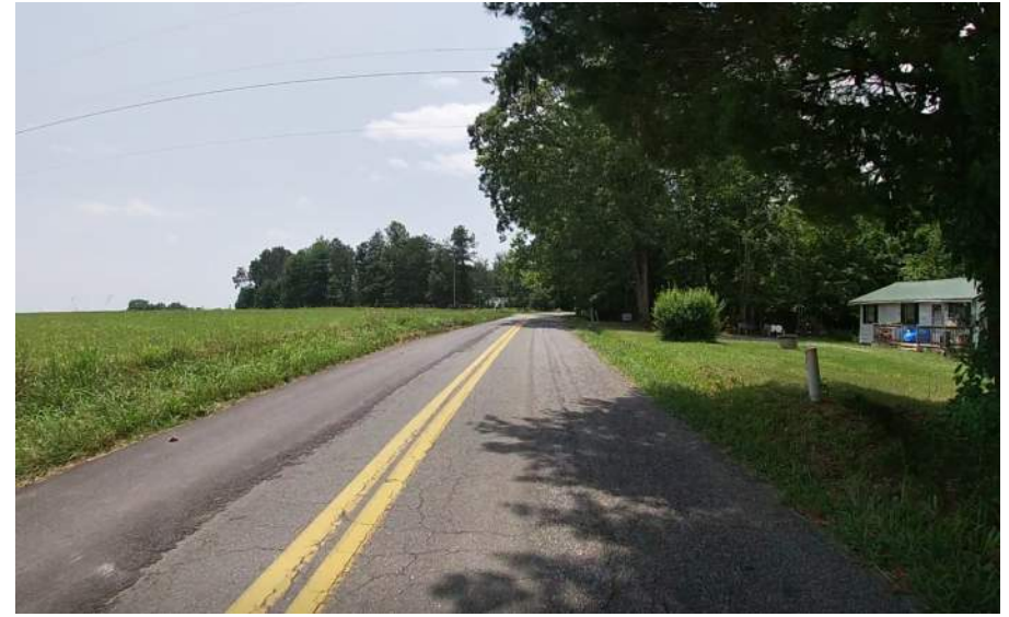
26. Block Cracking, Patching
