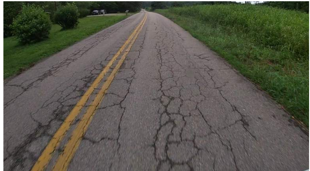
7. Block Cracking
