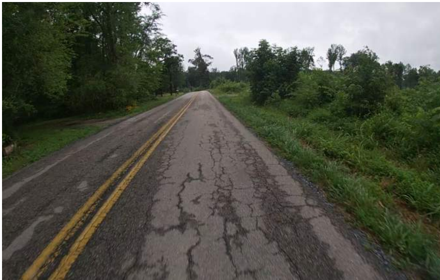
11. Alligator Cracking
