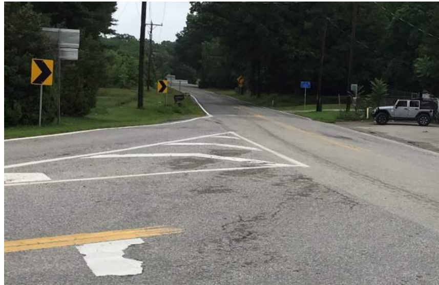
East along Route 45
