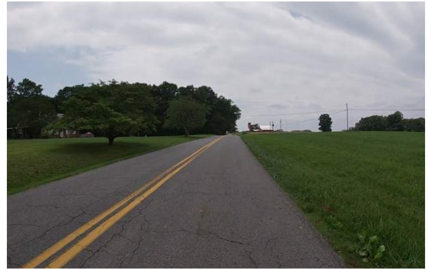
34. Block Cracking
