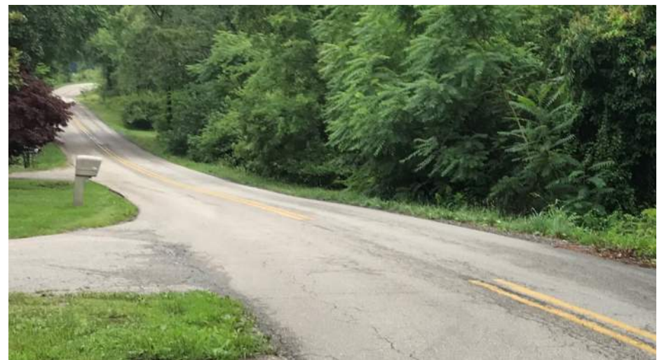
East along Route 690
