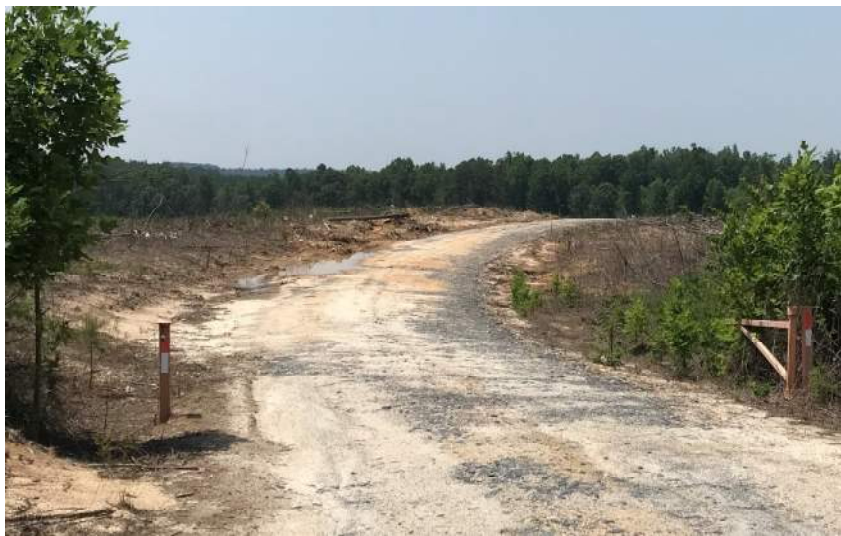
South along Site Entrance
