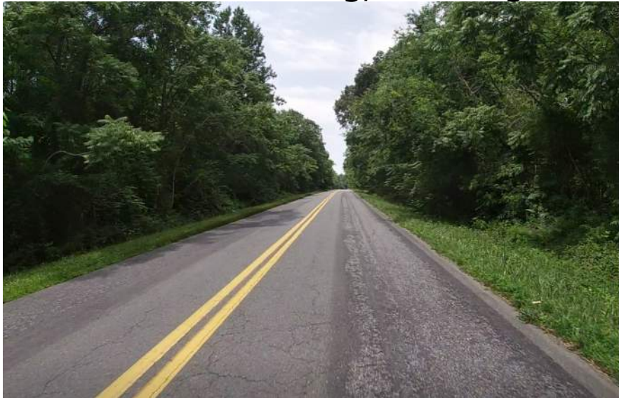
17. Block Cracking, Patching
