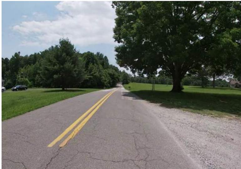
29. Block Cracking
