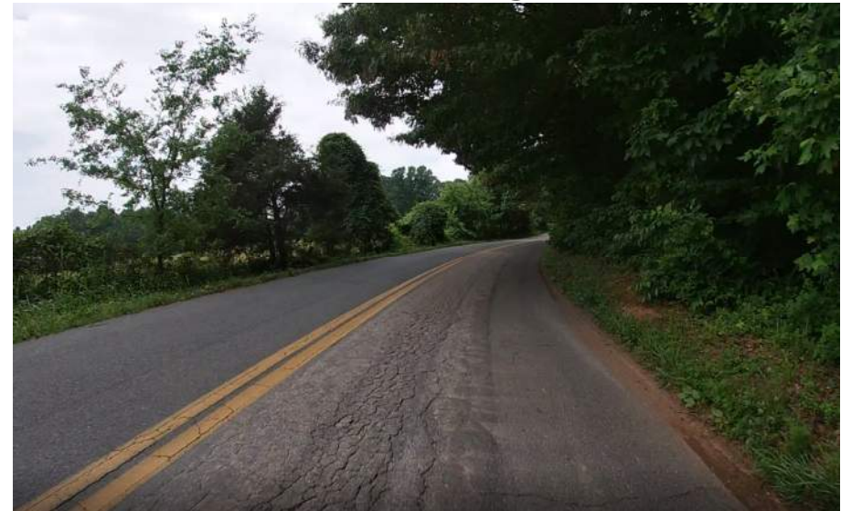
46. Alligator Cracking
