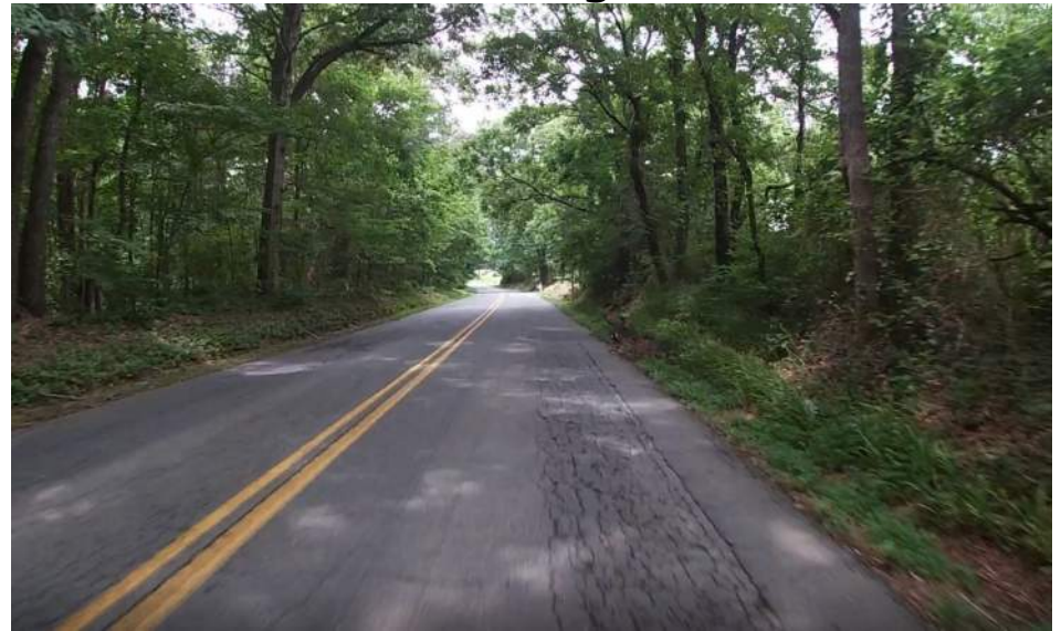
50. Alligator Cracking
