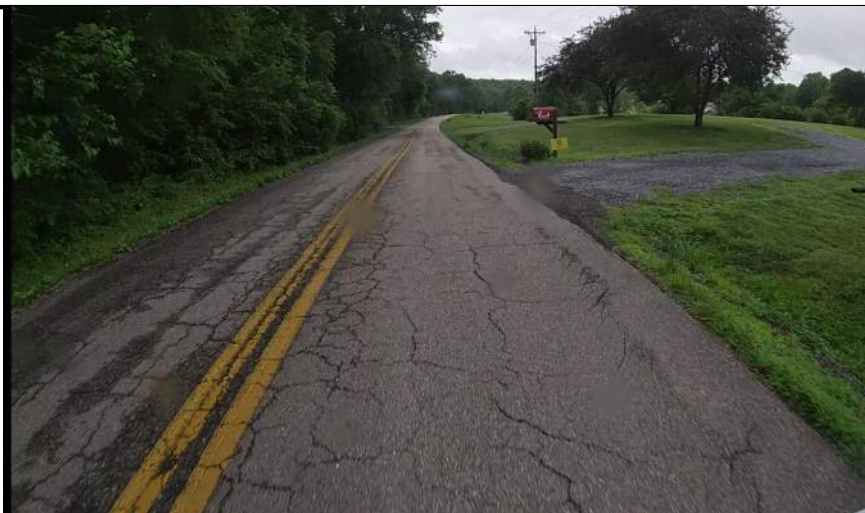
15. Alligator Cracking
