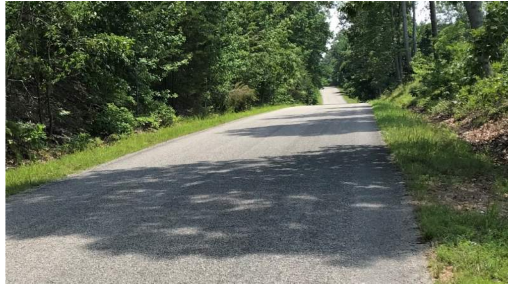
East along Route 609
