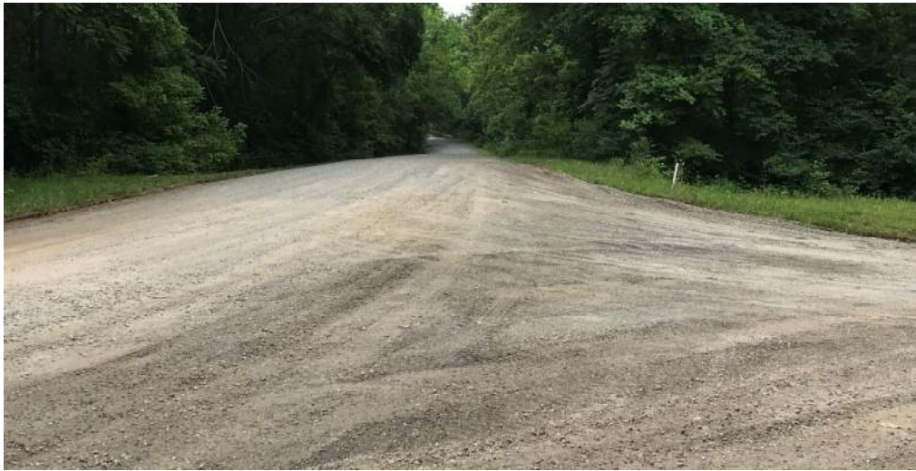
East along Route 608
