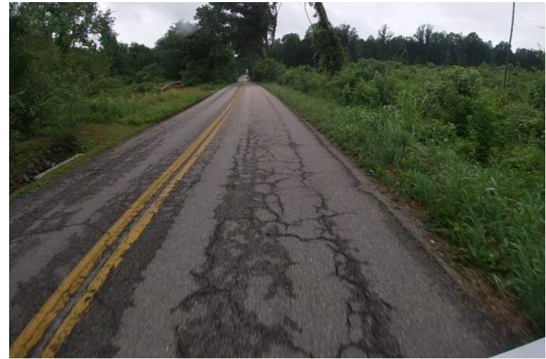
12. Alligator Cracking
