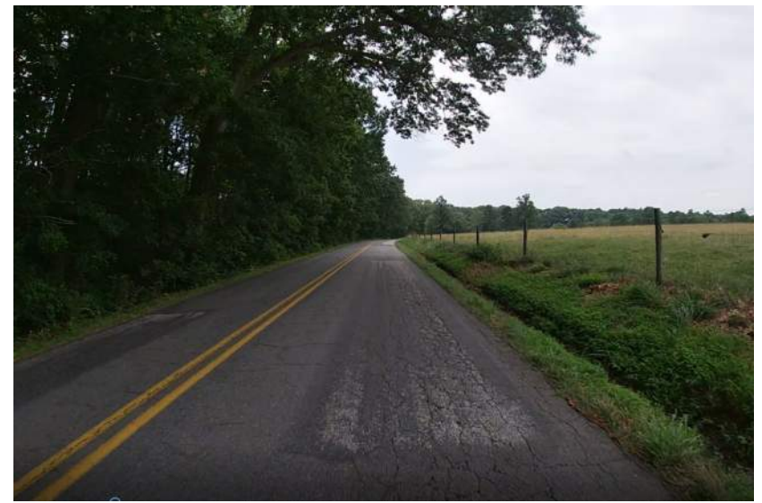
40. Alligator Cracking
