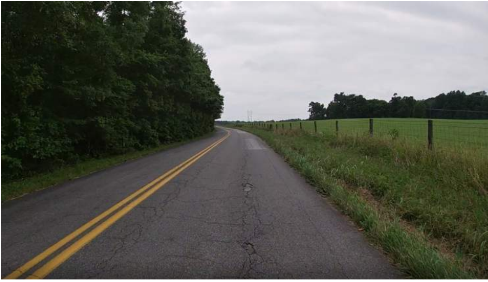
31. Alligator Cracking/Potholes
