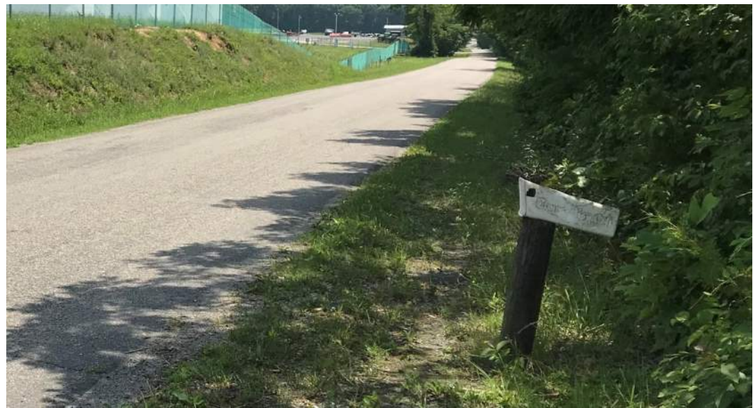
East along Route 609
