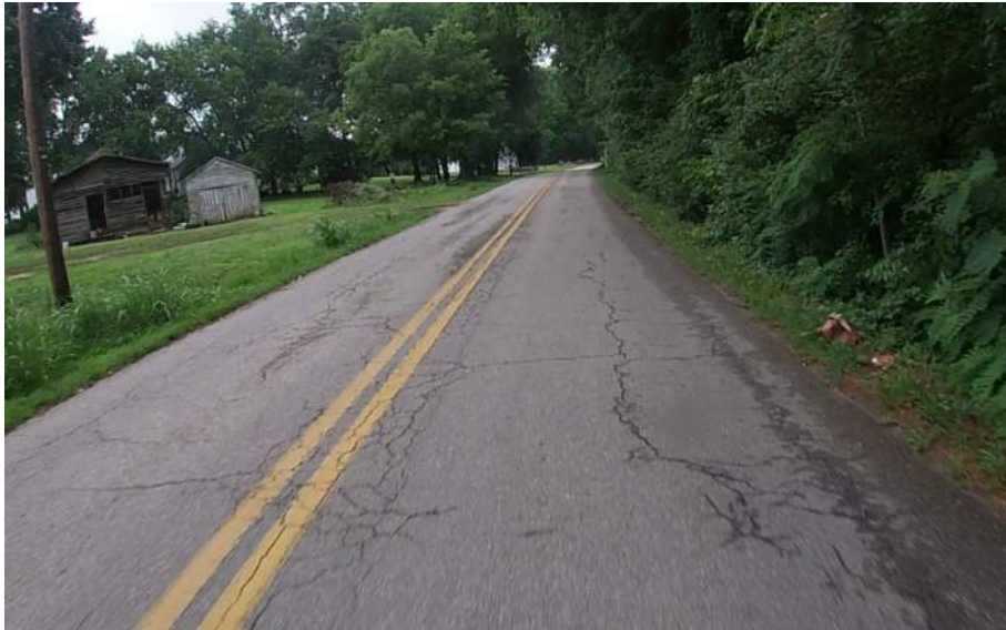
1. Block Cracking
