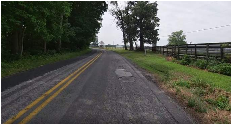
35. Patching, Alligator Cracking
