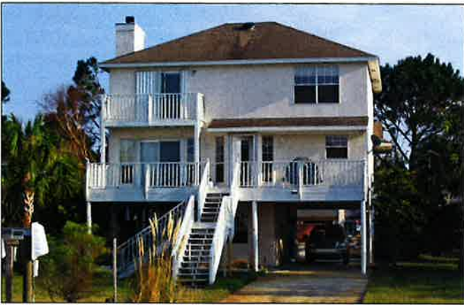
Elevated home on pile foundation
