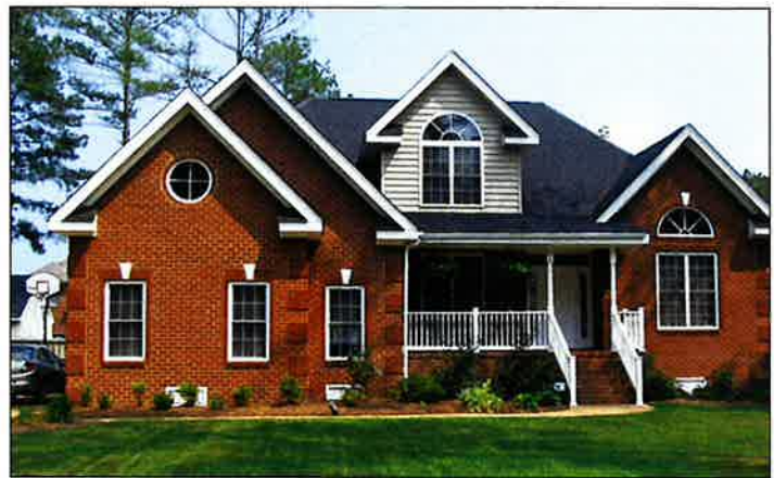
Elevated home on crawl space foundation
